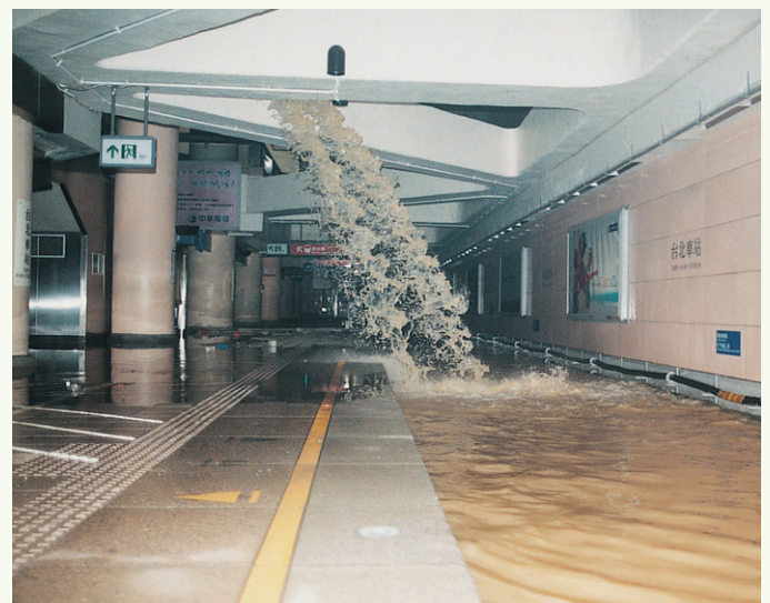
► Typhoon Nari caused serious damage to MRT.
